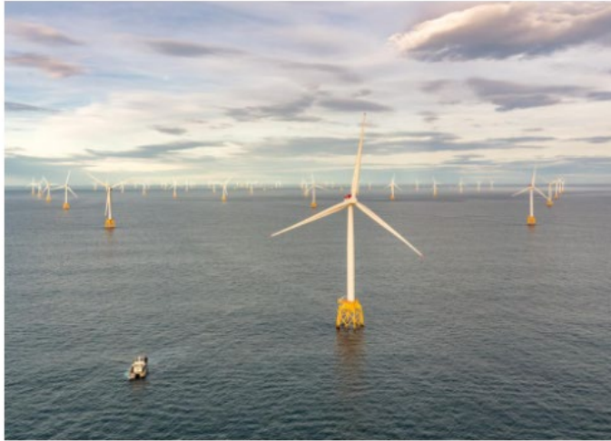
The proposed development will comprise 76 offshore wind turbines. FILE PHOTO
